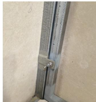
The rear panel (CR) has a notch on each edge and also slides under the tabs on the floor base (CB).
