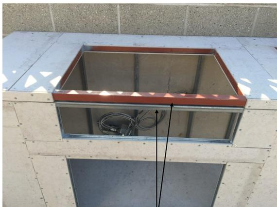
Front and Grill top panel prior to cutting. These front bars will always need to be cut regardless of grill size.
