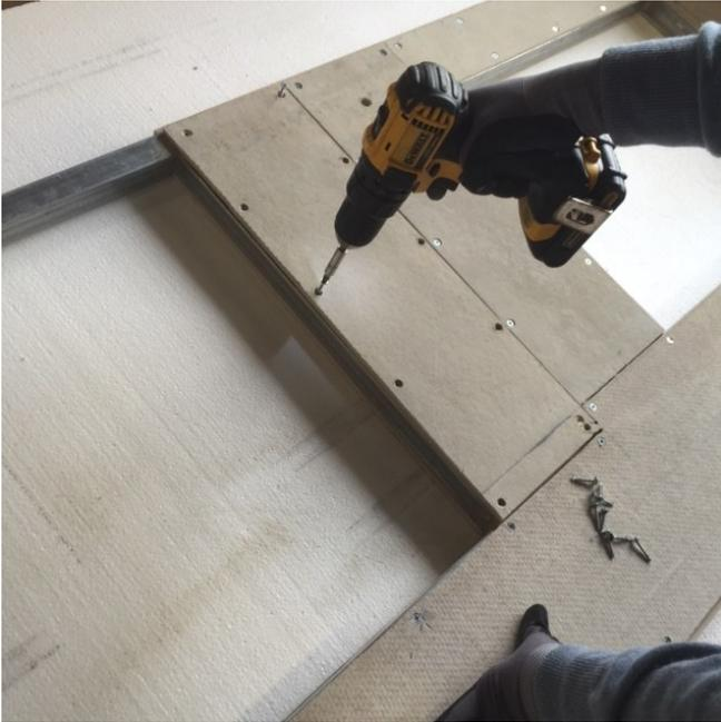
Remove the screws on the side panels
